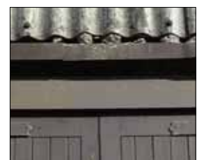
There could be sprayed limpet under this asbestos cement (AC) sheeting
